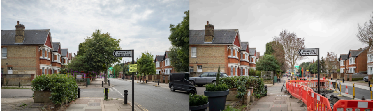
View 3 from Old Actonians Sports Ground of proposed block (full rendered and arrowed) cumulatively with other consented schemes (coloured red and purple):
