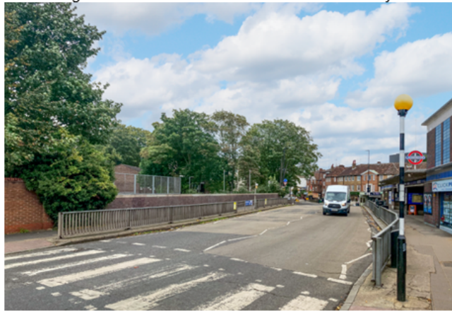
Existing view of south side of site from Gunnersbury Lane:
